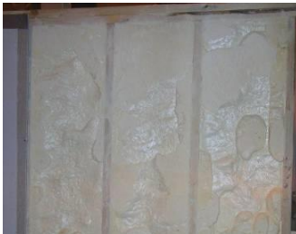
Slightly Underfilled Cavity
